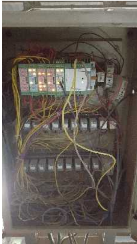
Gambar.2 Panel Radio Link sebelum upgrade
