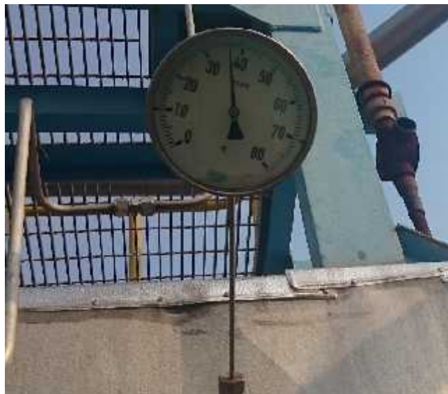
Gambar.1 Temperatur air pompa brine blowdown
