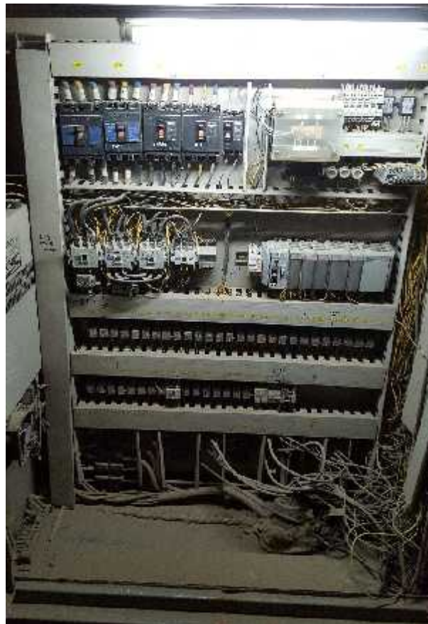
Gambar.1 Panel Kontrol sebelum upgrade
