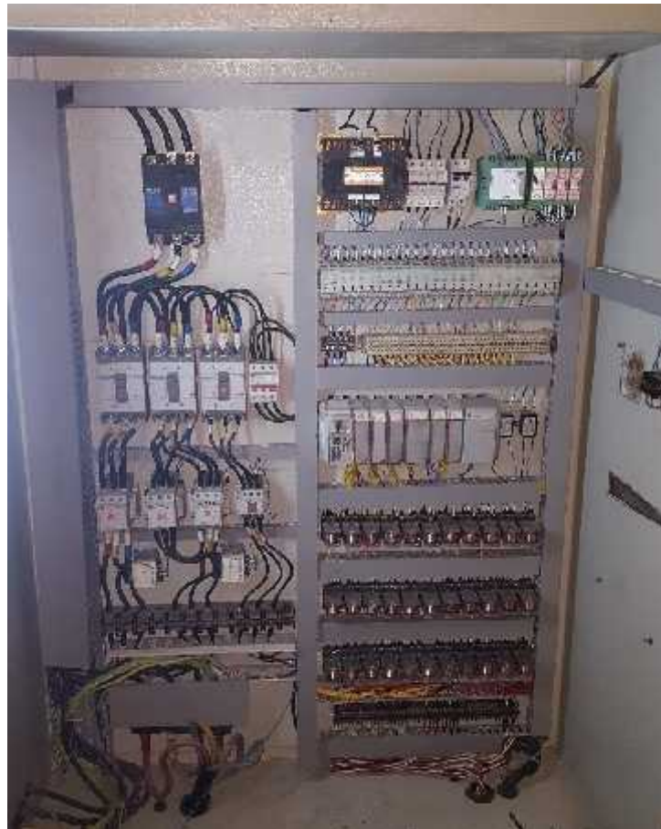
Gambar 3 Panel Kontrol setelah upgrade
