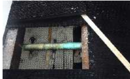
Gambar 3.19 Hasil Observasi Drift Eliminator Cooling Tower Sumber: PLTP PT. PGE Kamojang Unit IV
