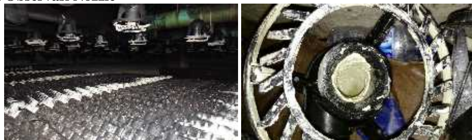
Gambar 3.18 Hasil Observasi Nozzle Cooling Tower
